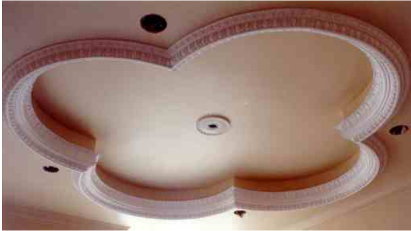
Ceiling Treatment including “Holly” Medallion , “Waterleaf Cutaway” crown moulding, and “Waterleaf Cutaway” medallion. Approximate Size: 9’ Diameter
